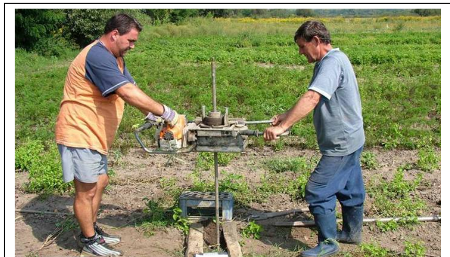
Figure 2: Shallow drilling, Galgahévíz, Hungary.
