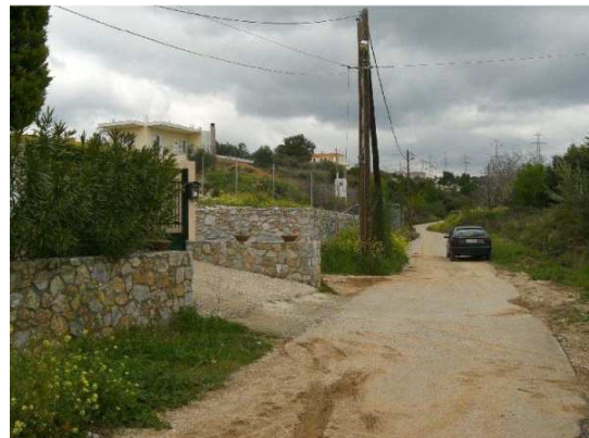
Fig.5: Roads and houses on streambeds (Source: Laskaris 2008)
