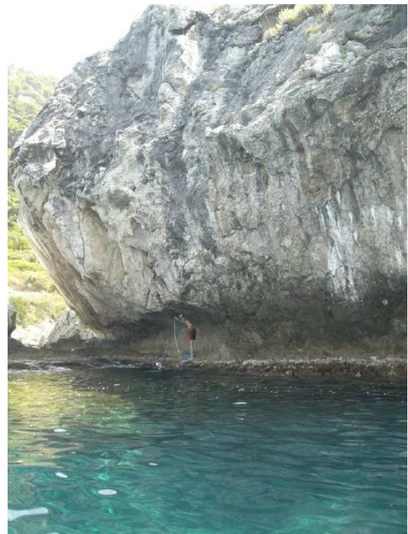
Figure 3. Shoreline B, emerged at +110 \pm 11 cm, is detected through an abrasion notch.
