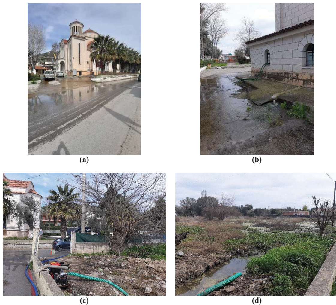
Figure 4. Periodical flooded area of the Church Ag. Eleousa; a: road in front of Church; b: pumping floodwater from church; c: pumping water from plot (d); and d: flooded plot
