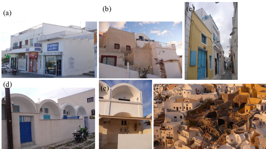
Fig. 6 a RC buildings; b simple stone buildings; c ground floor in stone and additional floors in RC frame; d post-seismic cement brick vaulted structures; e mixed buildings with brick-cement vaults at the ground floor and overlying RC frame; f excavated dwellings
