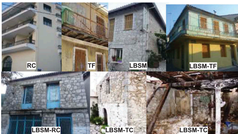
Figure 4. Examples of the Lefkas buildings typologies. Photos taken by our group in 2015–2016 and Kalantoni [2016].
