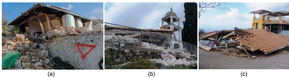
Figure 15. (a) Red tagged LBSM-TC building in Dragano with successful performance of TC frame (b) Collapsed Agia Paraskevi church in Athani; (c) Collapsed kiosk near Athani.
